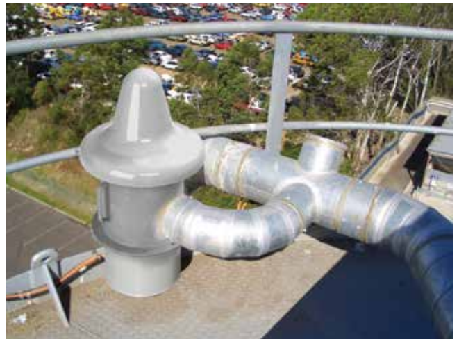
VHS Pressure Relief Valve releasing excess pressure
